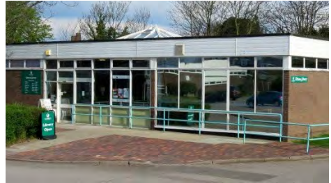
Dittons Library at Mercer Close
