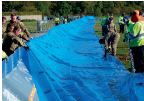
Demonstration of a temporary flood barrier
