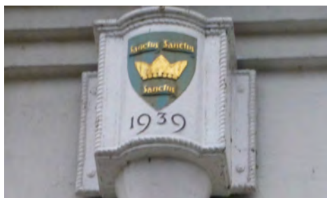
Downpipe with a differencer
