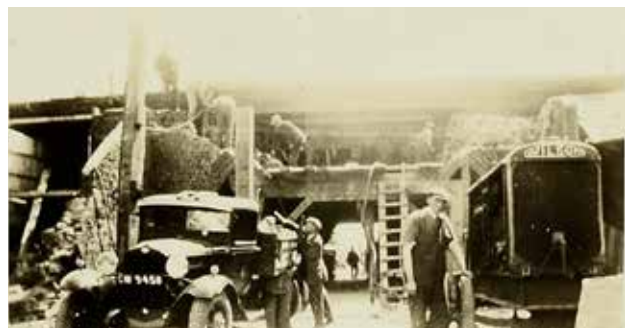
1931 Construction of the new railway bridge for Hampton Court Way at Tuckers Arch.
