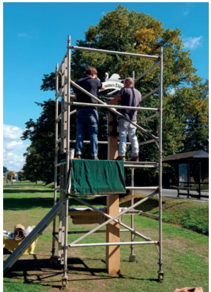
Erecting the new village sign
