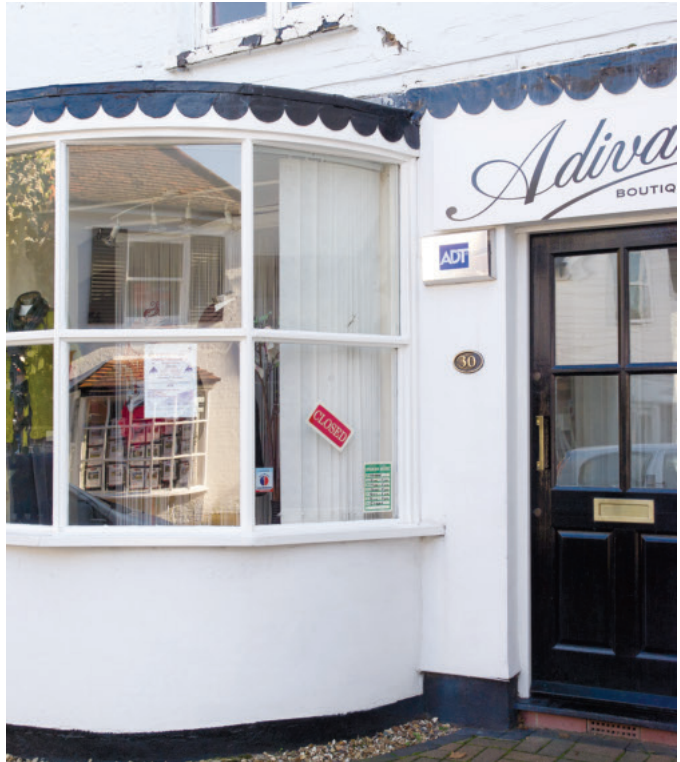
protection for this attractive shop would be lost
