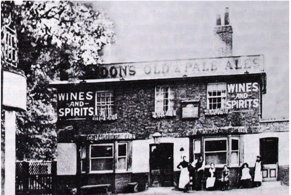
the former Olde Harrow, altered since Georgian times, before demolition in 1905 and replacement by the present doomed building
